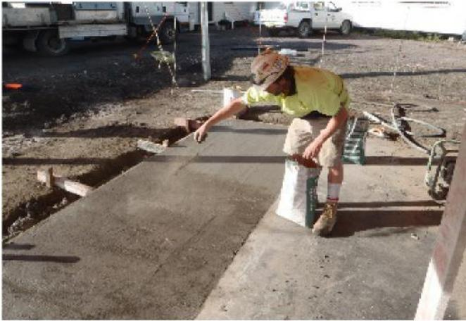
**Figure 8: Fill in the areas which have less shake**
