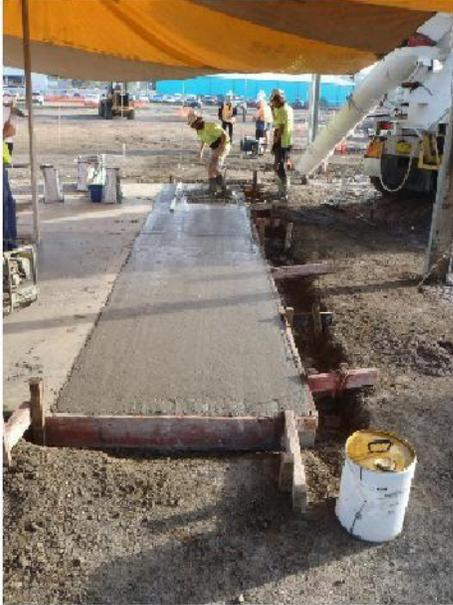
**Figure 1: Screeding the concrete**
