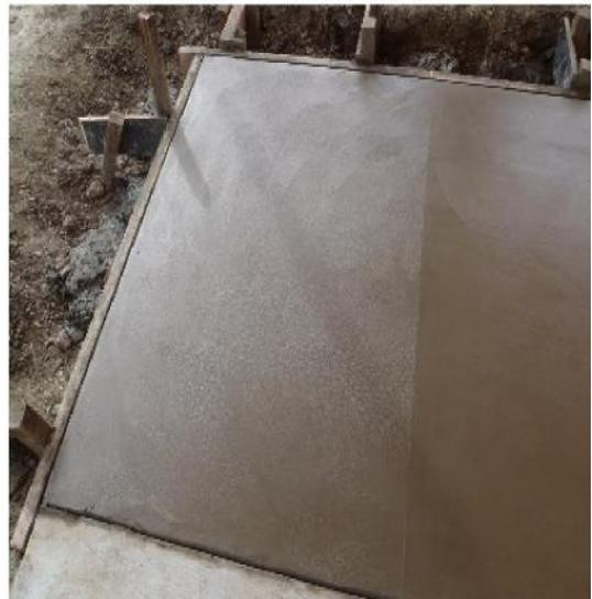
**Figure 16: finished floor prior to curing.**
