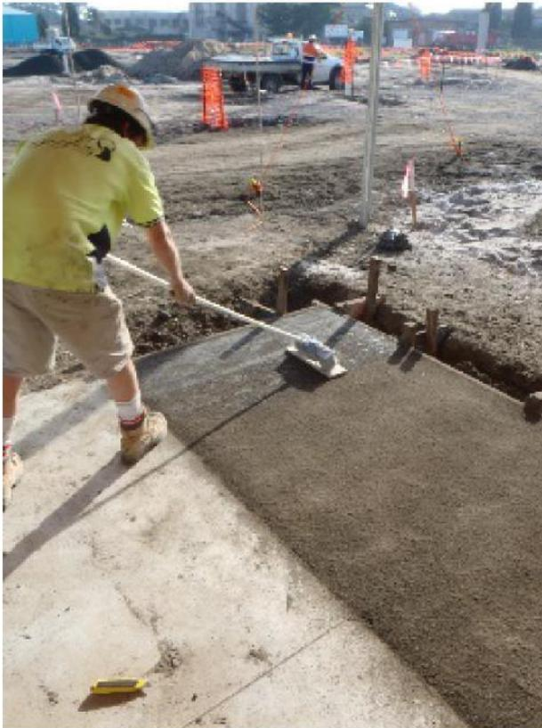
**Figure 11: Using a bull float to flatten and bring the moisture to the surface.**
