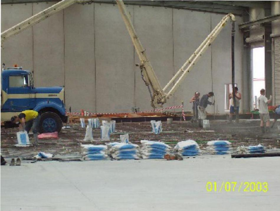
**Figure 17: set out bags prior to delivery of concrete**
