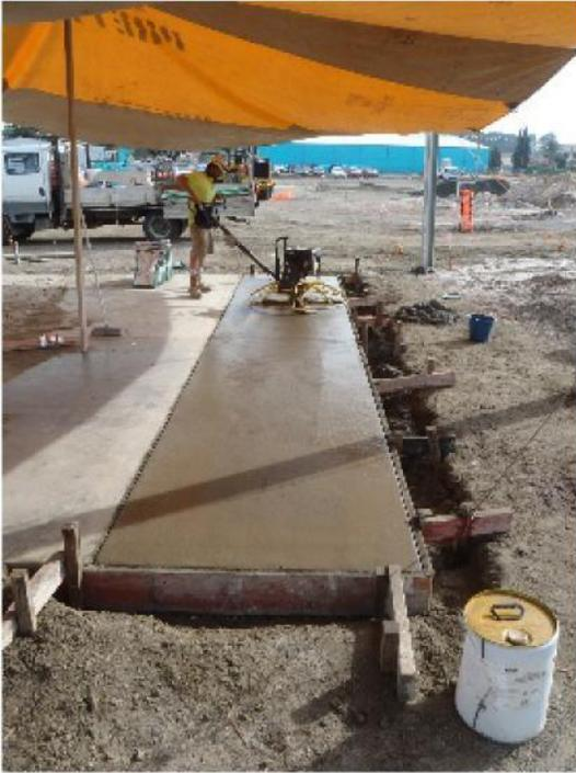
**Figure 13: after bull floating power trowel the shake**
