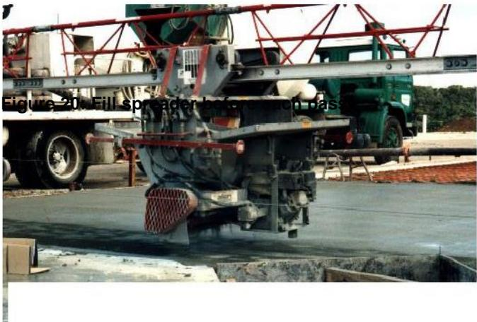
**Figure 21: Spreader applying the shake**
