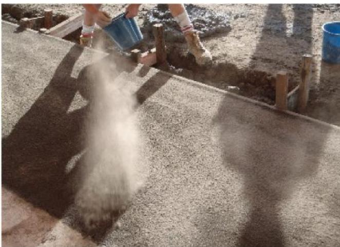
**Figure 9: apply using the "feeding the chooks" method**
