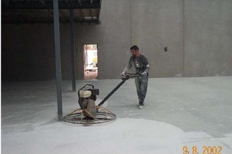
Figure 24: Once the concrete will not be marred use the helicopter to smooth the shake
