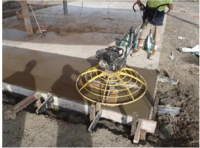
**Figure 14: Keep the blades flat to consolidate the shake**
