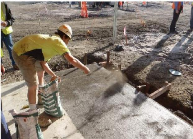
**Figure 5: Allow the shake to fall onto the surface from above**
