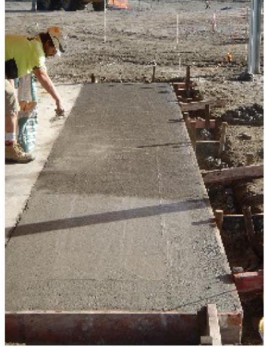
**Figure 4: See how the shake soaks up the moisture from the fresh concrete**
